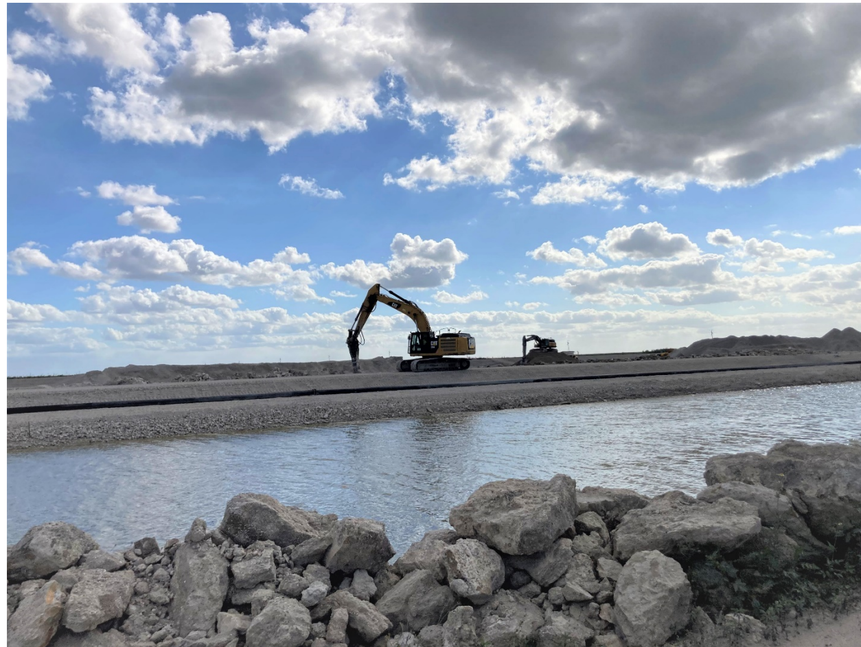
Inflow/Outflow Canal and Levee Construction
