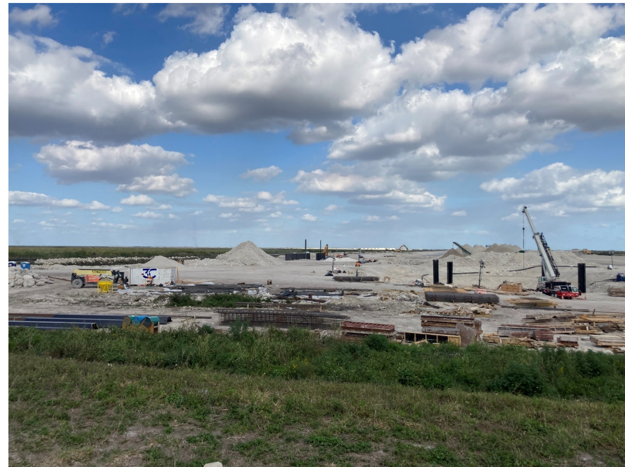
S647 Spillway Structure & S648 Seepage Pump Station
