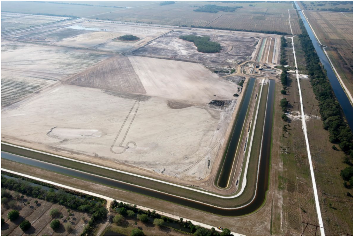
C-23/C-24 Stormwater Treatment Area Construction, APR 2023
