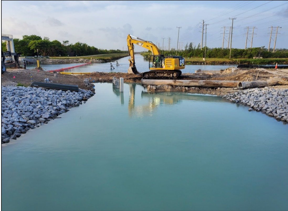
S-705 Construction Site
